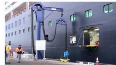
Cable support beam on quay
